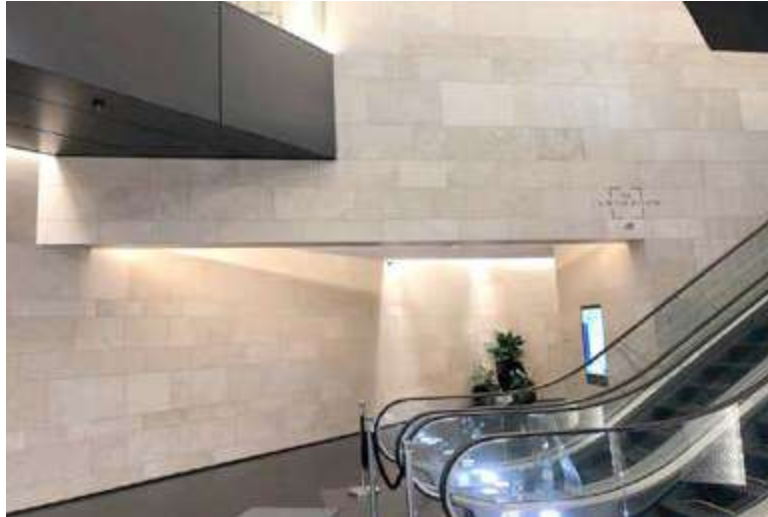
45 Queen Street Prada and Dior Cladding Auckland - NZ
