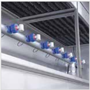
Series of nozzles for water nebulization.
