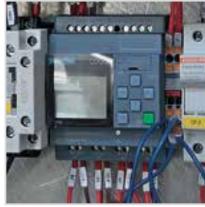
PLC to program times and modes of automatic cleaning.
